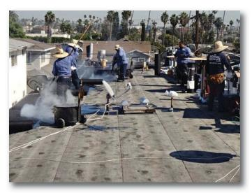
roof, and its seams melt together to create a waterproof seal.
