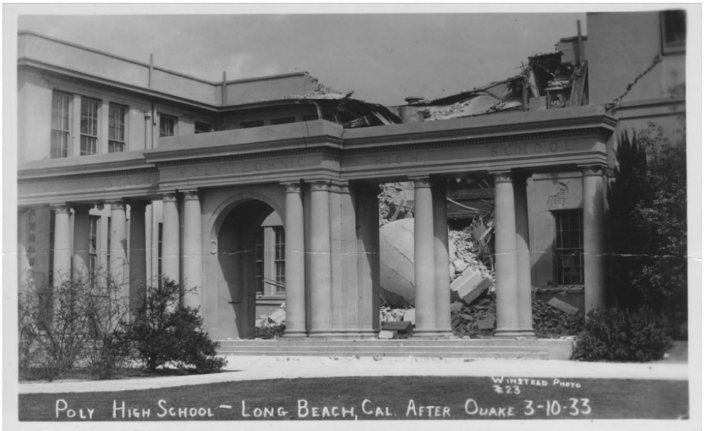
Most of the Poly High School campus was destroyed in the earthquake, but the auditorium survived. (Source: Loyola Marymount University)
